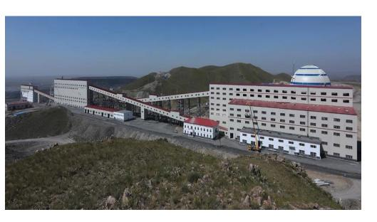
Newly completed 30,000 tpd crushing system
