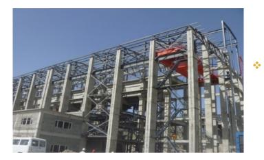
Crushing workshop: steel body and platform completed, four cone crusher bases are in place.
