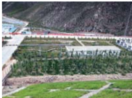
Vegetation around the plant
