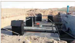
Construction of waste water treatment station
