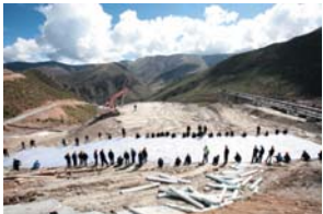
Treatment on tailing dam
