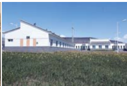
Vegetation around the dormitory
