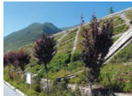
Slope Protecting and Greening
