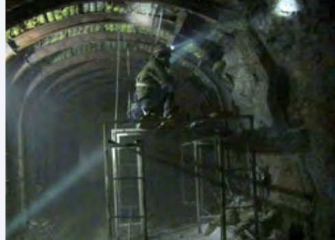
Jiama Mine conducted danger removal inspection on pumice stone
