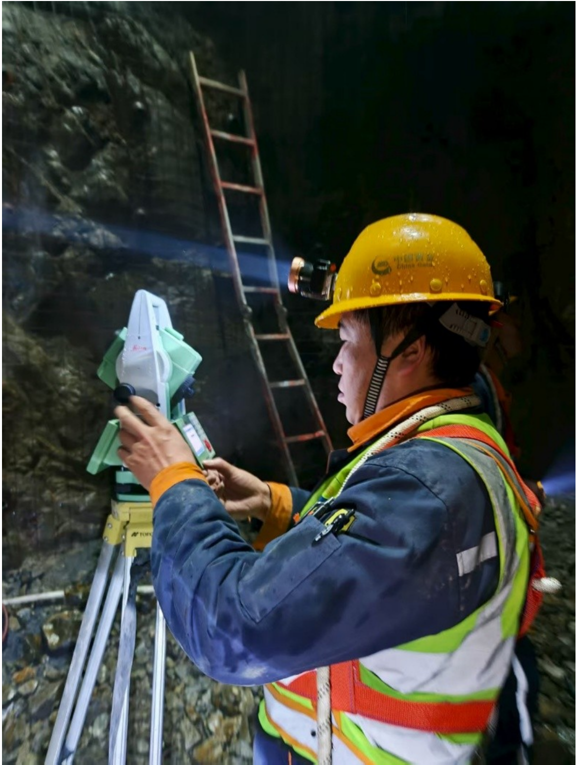
Figure 10. 3 Collar Survey During Underground Drilling
