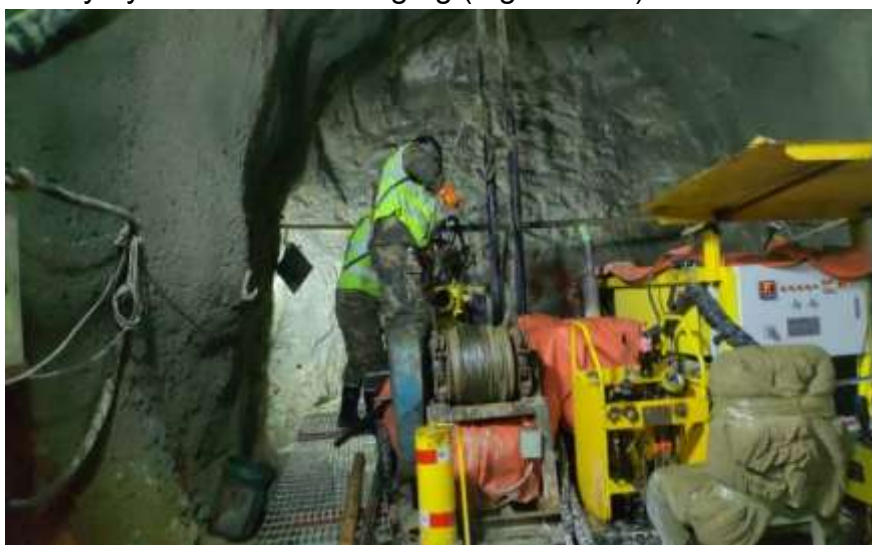
Figure 10. 4 Underground Drill Rig
