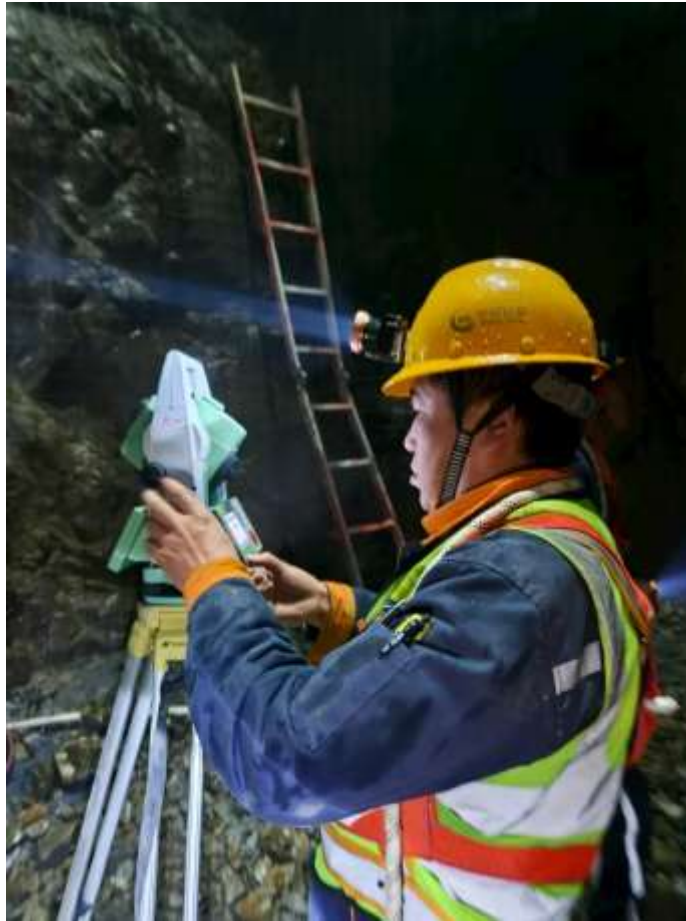
Figure 10. 3 Collar Survey During Underground Drilling
