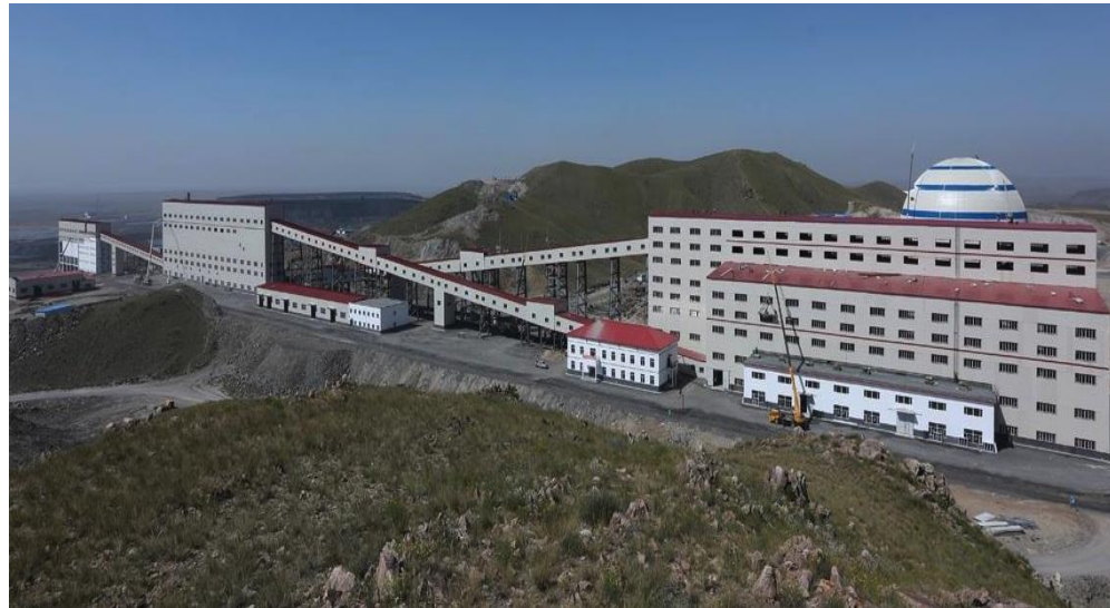
Newly completed 30,000 tpd crushing system
