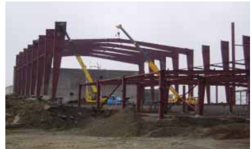
Construction of Gold Process Plant
