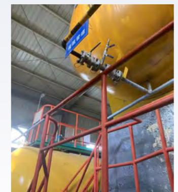
Liquid cyanide pipeline valve of liquid cyanide warehouse after rectification
