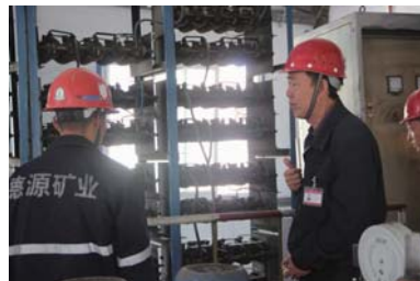
Personnel of Huatailong were inspecting winch room area of 4620 inclined shaft.
