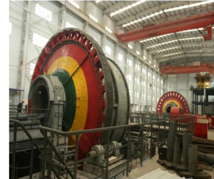
❖ major equipment installed
