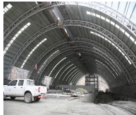
❖ construction of ore storage
